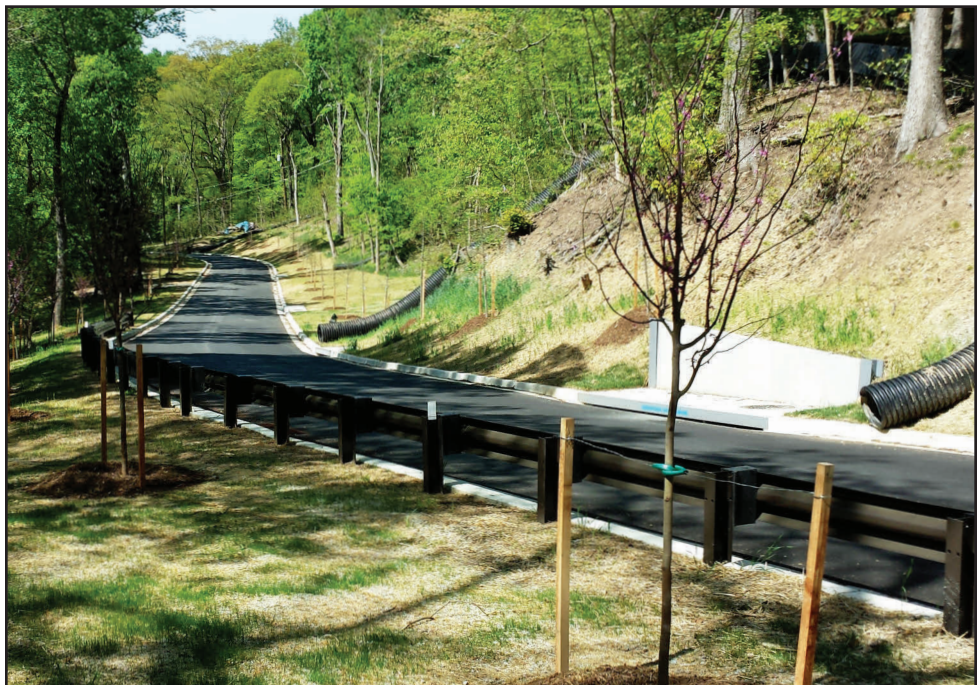
2017 GRAND AWARD KCI Technologies Inc. Piscataway Hills Landslide Stabilization
