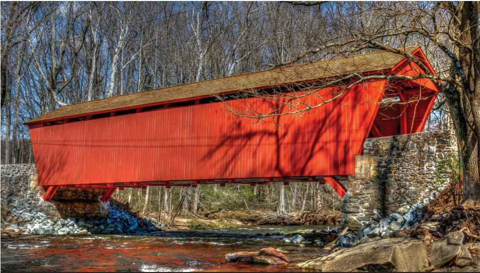
Wallace Montgomery Jericho Road Historic Covered Bridge Rehabilitation
