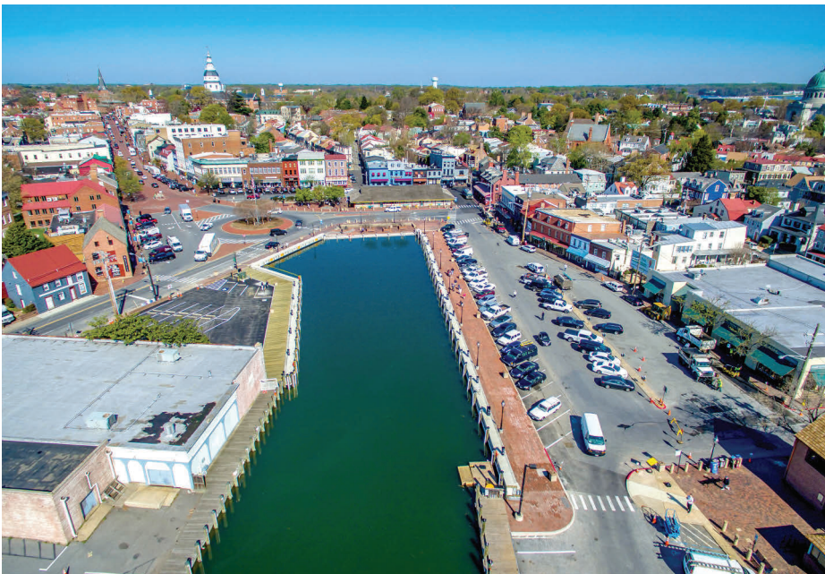
EBA Engineering Inc. Annapolis City Dock Bulkhead Replacement Phase 2
